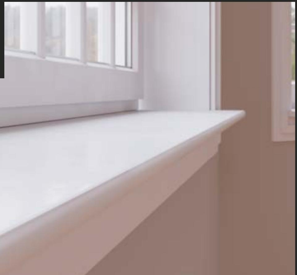
The MDP and MDF Bullnose Mouldings application are a specialized use of Medium-Density Particle board or Medium-Density Fiber board bullnose mouldings, which are a versatile and popular trim material used in various architectural and interior design projects. Bullnose mouldings are specifically designed with a rounded or curved edge, commonly referred to as a bullnose profile.
